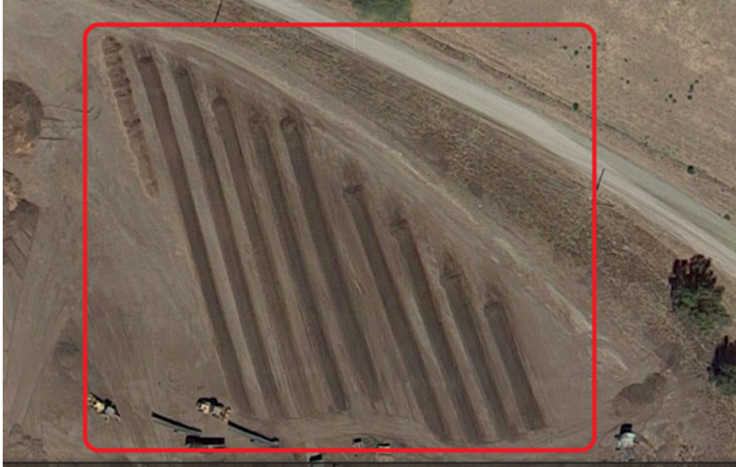
Figure 1. Compost Facility on Cal Poly Campus, CA (Google Maps. 2015)
