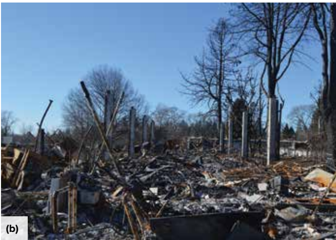
Fig. 9: Remains of buildings destroyed in the Camp Fire: (a) Stratton Market; and (b) Paradise Elementary School (photos courtesy of Erica Fischer)
