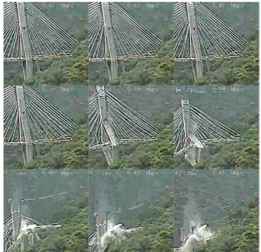
Fig. 8: Chirajara Bridge west tower failure sequence (after Reference 29)
