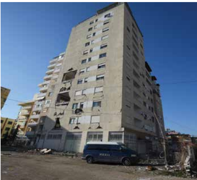
Fig. 10: A damaged mid-rise RC-frame building in Albania
