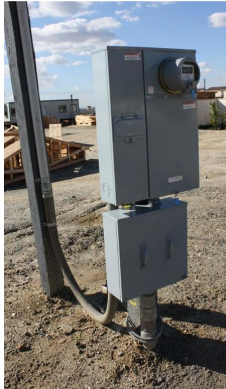
*Figure 1* – Typical established temporary power connection and panel with meter and shutoff box
