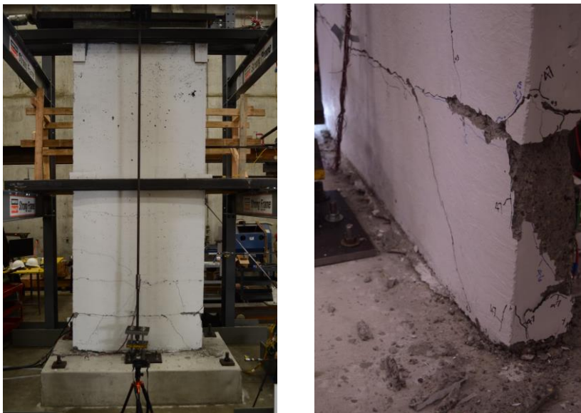
Figure 6. Final damage state of wall: (left) overall, (right) north wall end zone
