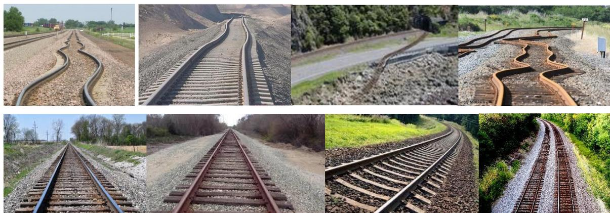
Figure 8. Input images for railways: (top) horizontal offset, (bottom) no horizontal offset.
