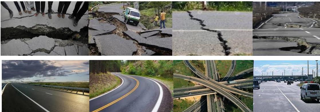
Figure 6. Input images for roadways: (top) cracking, (bottom) no cracking.
