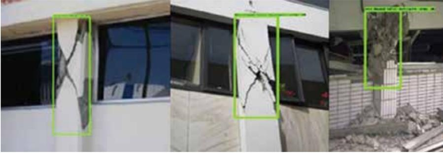
**Fig. 6: Bounding box classification results: shear damage to short/captive column**
