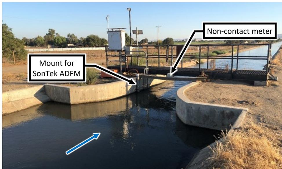
**Figure 1. PID Main Canal subcritical contraction structure with non-contact meter installation and SonTek ADFM**
