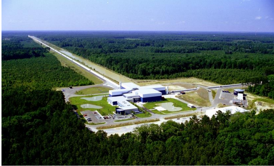
Figure 1: A picture of the LIGO Livingston site with the two perpendicular arms that extend for 4 kilometers.
