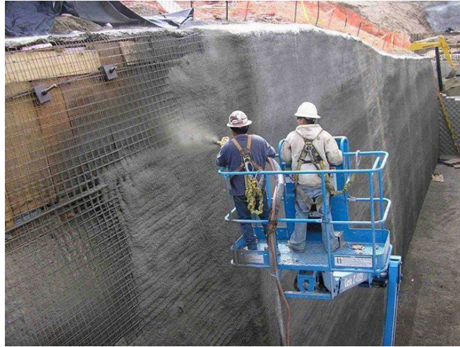
Figure 5 – Shotcrete Application on Commercial Foundation
