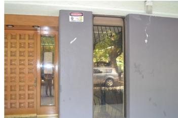
LEFT: 55 AVE. MEXICO: CONCRETE CORE WALL SURROUNDING STAIRWELL (DARKER AREAS INDICATE POXY ADDED AFTER 1985 EARTHQUAKE)
