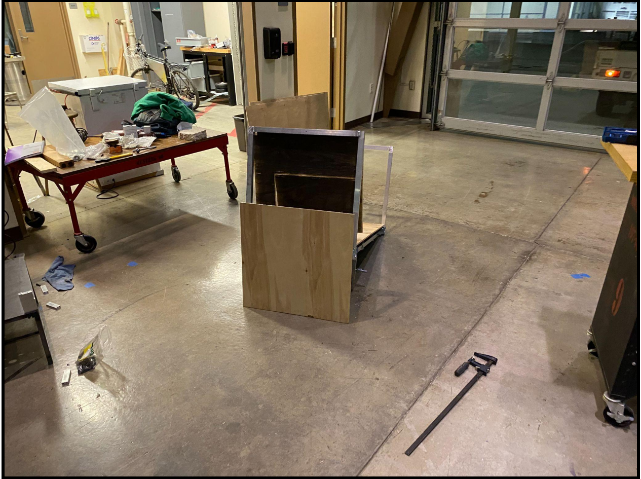
Mounting the plywood walls
