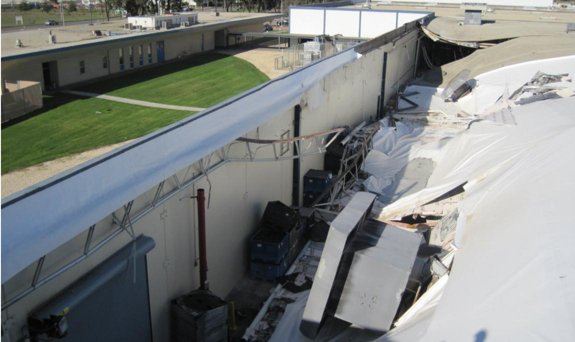
**Figure 1 - Excessive rainwater load causes a steel roof structure to collapse.**
