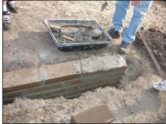
**Figure 5:** Brick wall laid directly on ground starting 5 course below grade
