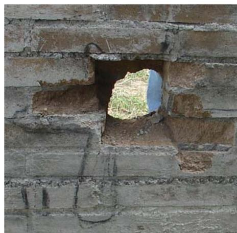
**Figure 14:** Double wythe wall and penetration, back face
