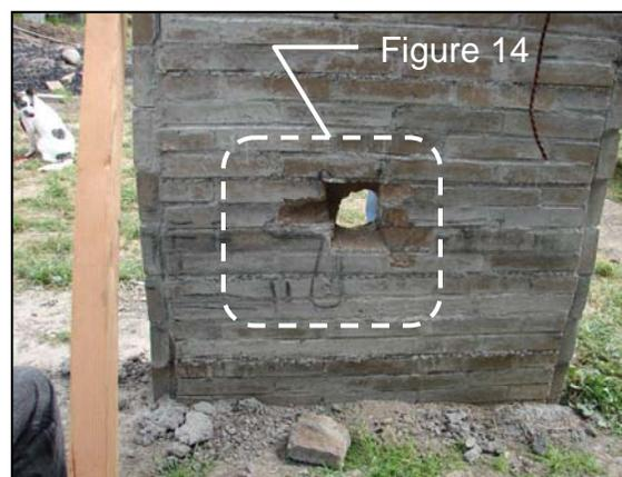
**Figure 12:** Double wythe wall and penetration, back face
