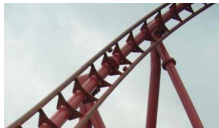
Fig. 1—Roller coaster track with circular backbone and rails.
