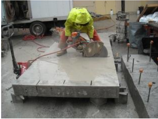
Figure 10: Cutting Wall 3 at Every Course with a 16” Diameter Diamond Blade Cut-Off Saw
