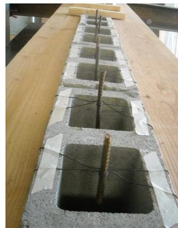
**Figure 6: Wall Construction (a) Horizontal Steel Placement and (b) Vertical Steel Placement**
