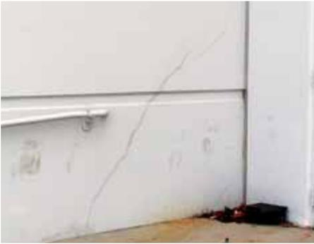
Figure 4. Cracking associated with base restraint.
