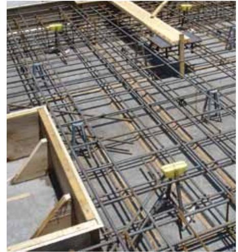
Figure 6. Diagonal corner bars to control cracking.
