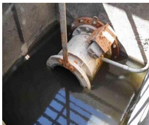
Figure 6. Magmeter located upstream to a farm turnout in Patterson Irrigation District (Styles, 2012).
