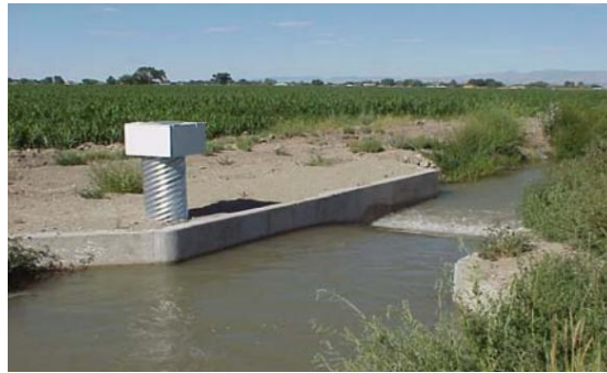
Figure 7. Replogle flume at Truckee-Carson Irrigation District (ITRC, 2002).
