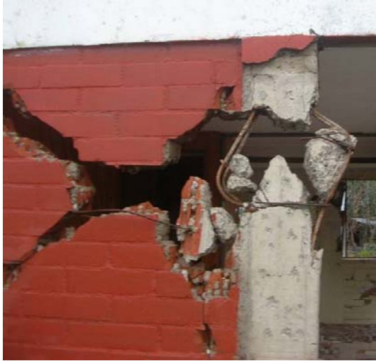
Figure 23. Buckling of longitudinal reinforcement due to inadequate confinement in the end zones of RC tie-columns (Brzev et al., 2010).
