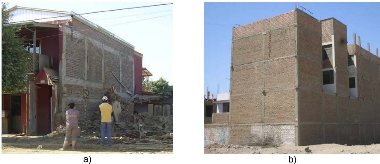
Figure 4. Performance of confined masonry buildings in recent significant earthquakes: a) the 2010 Maule, Chile earthquake (M.O. Moroni Yadlin), and b) the 2007 Pisco, Peru earthquake (D. Quiun).
