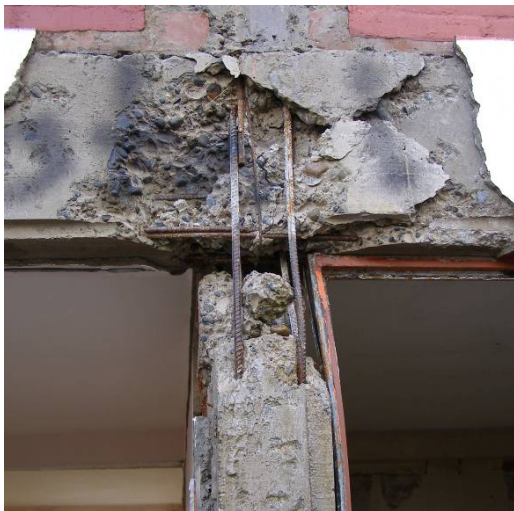
Figure 23. Buckling of longitudinal reinforcement due to inadequate confinement in the end zones of RC tie-columns (Brzev et al., 2010).
