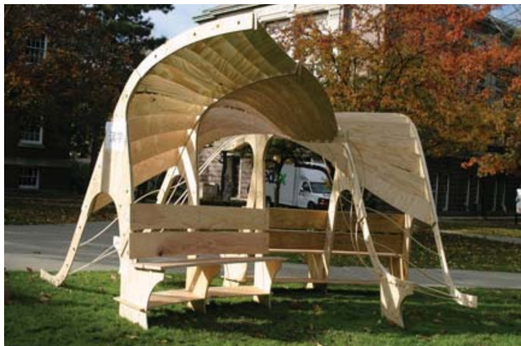
Full Scale Sketch Model? This team quickly modeled the vertical ribs, but believed their digital model rather than testing joints or the way they assumed materials would bend. ▲
