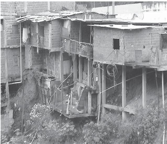
*Figure 1. An example from Caracas , Venezuela, of how unstable self-built housing can be. (photo by W. Siembieda)*
