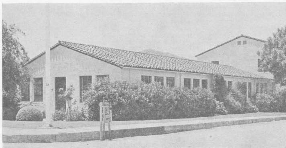
Air Conditioning Building
