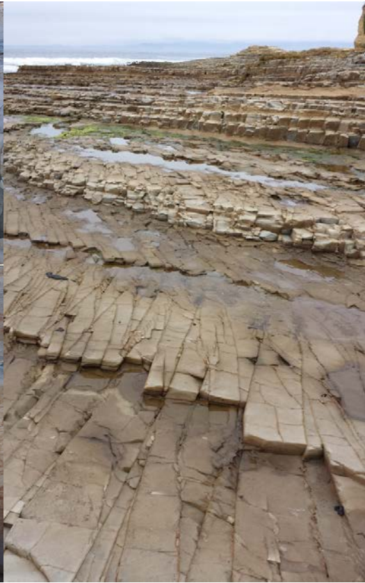
Image 2. Example of a conjugate joint system located 1 km south of Hazard Canyon.
