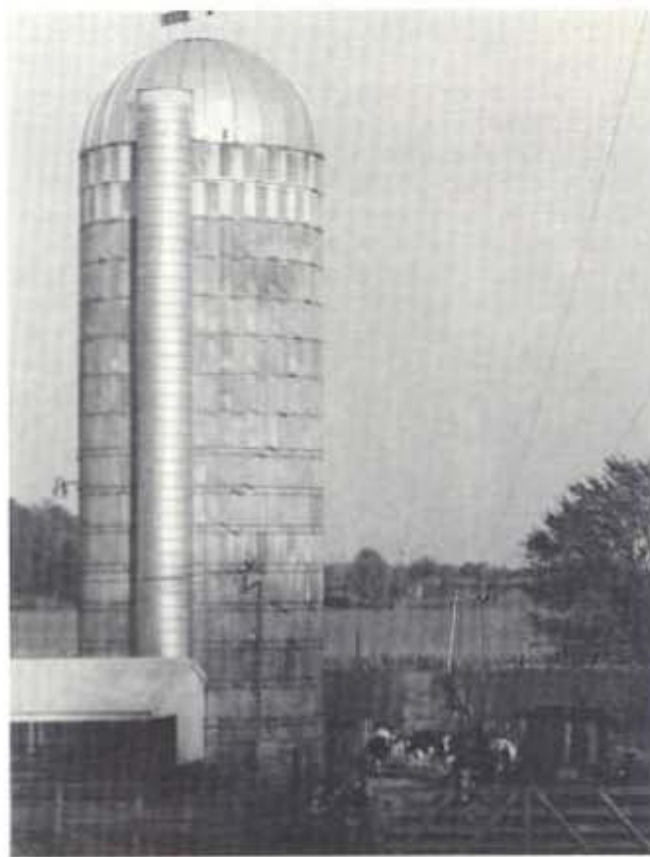
Figure 5: Concrete stave silo.
