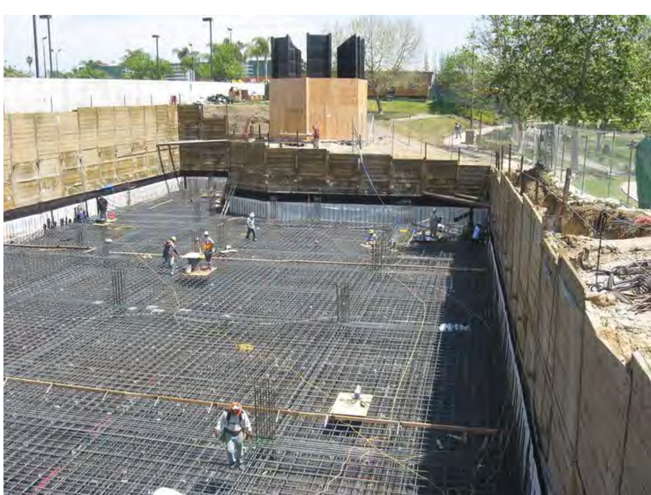
Example of Mat Foundation Construction
