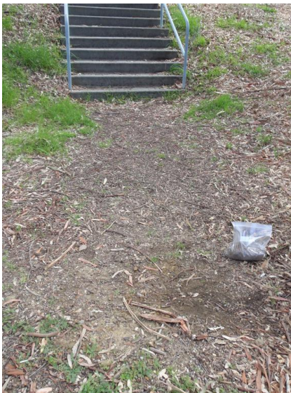
Figure 9. Footpath and staircase behind red brick dormitories
