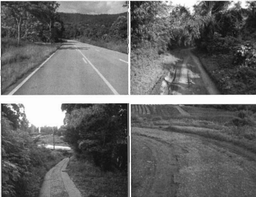
Figure 4. Various road conditions measured in this study.
