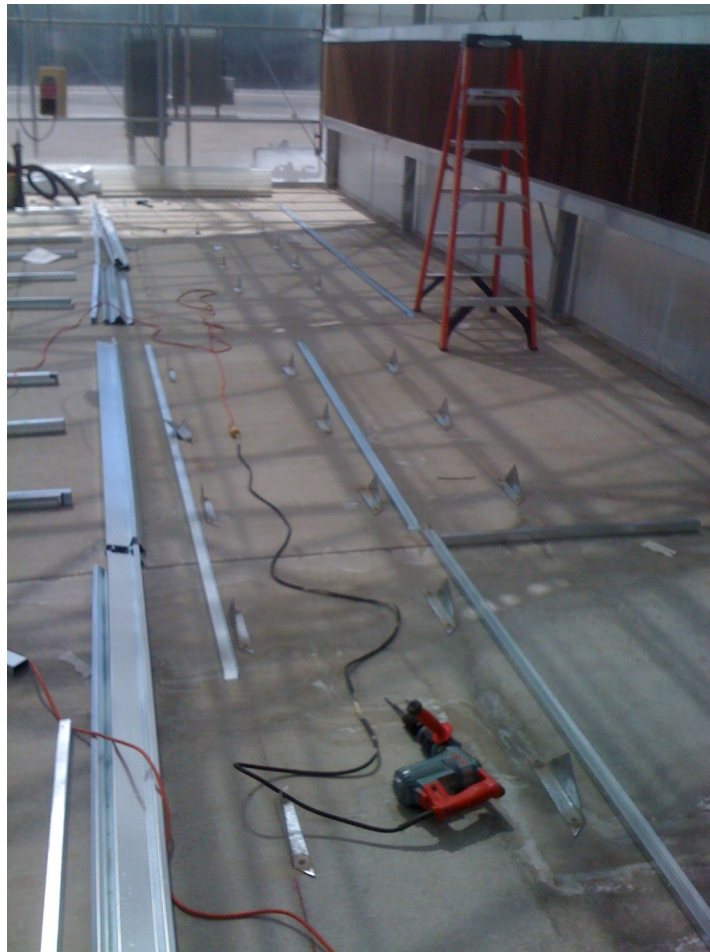
FIGURE 3. Beginning of Bench Construction
