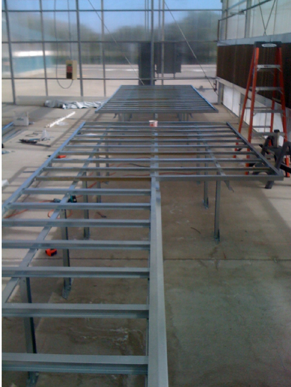
FIGURE 4. End of Bench Construction I
