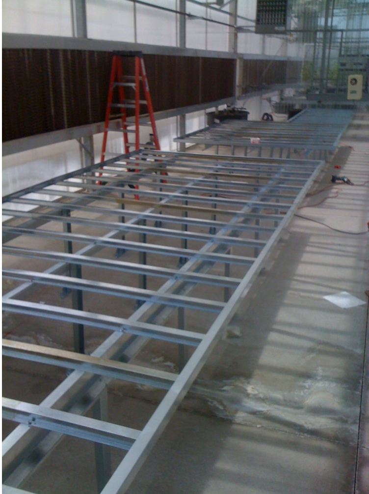
FIGURE 5. End of Bench Construction II
