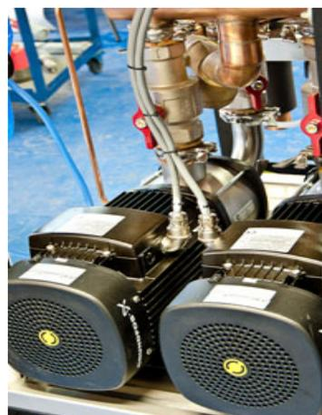
Figure 4. Redundant Pumps in CDU
