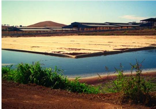
Water from the wastewater ponds is pumped to giant water cannons for distribution onto campus pasturelands. By applying the water to the soil, nutrients, pathogens and sediments are removed and the groundwater is recharged.
