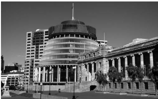
The national government center in Wellington, also known as "beehive". (Photo: P. Wack)
