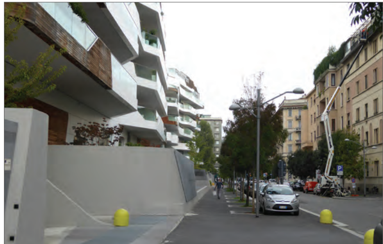
Figure 2: Designed by Zaha Hadid, residential buildings in Milan, fails to respond to Milan’s 19th century fabric.
