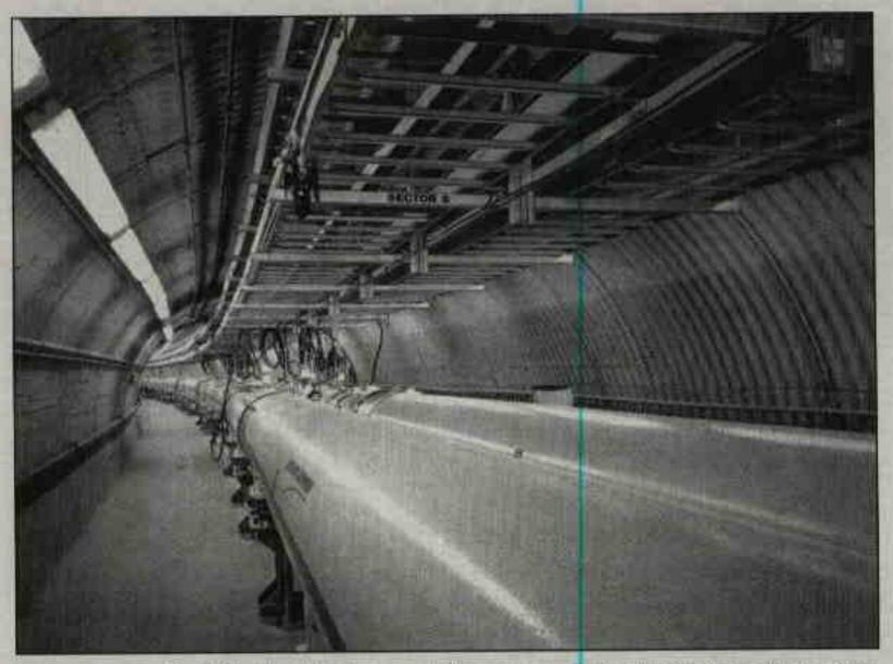
RHIC magnets, a view inside the RHIC ring tunnel. Photos courtesy of Brookhaven National Laboratory.
