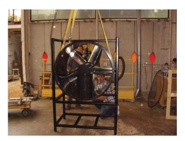
Figure 8. Installation of fan in motor stand.
