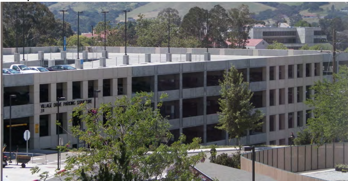
Figure 4.3 – 3: Unscreened parking structures are generally unappealing visually.
