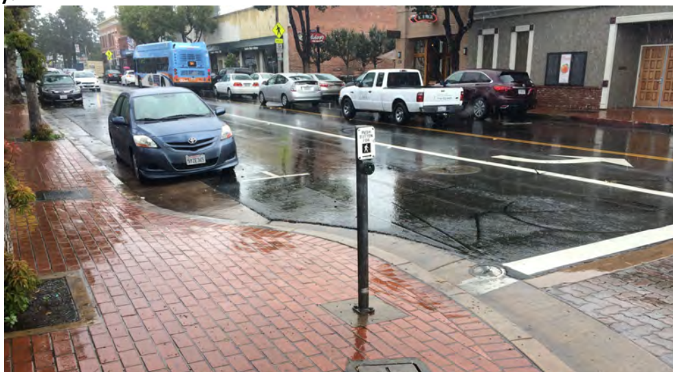
Figure 4.4 – 10: While benefitting pedestrians, bulbout features also improve traffic safety by requiring vehicles making right turns to slow down around a sharper turn radius.
