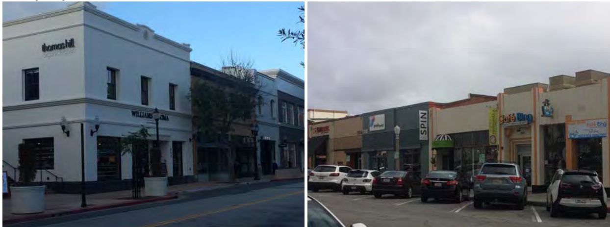
Figure 4.2 – 13: These neighborhoods benefit from having an overall aesthetic goal. The new buildings complement the existing ones, generally creating a seamless fabric when viewed as a whole.
