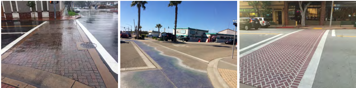
Figure 4.4 – 11: Various techniques involving color and texture can be used to increase the visual prominence of crosswalks. Pavers (left), textured paint (center), and concrete treatments (right) all stand out better against the street compared to traditional striped crosswalks.
