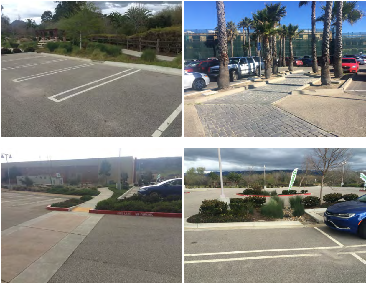
Figure 4.3 – 7: Parking lots should adequately consider connections between the parking area and the main corridor with prominent sidewalks and crossings (top right, bottom left). Surface parking should also incorporate landscaping (top left, top right, bottom left, bottom right) to maximize greenspaces citywide, and incorporating bioswales to minimize storm water runoff (top left, bottom right).
