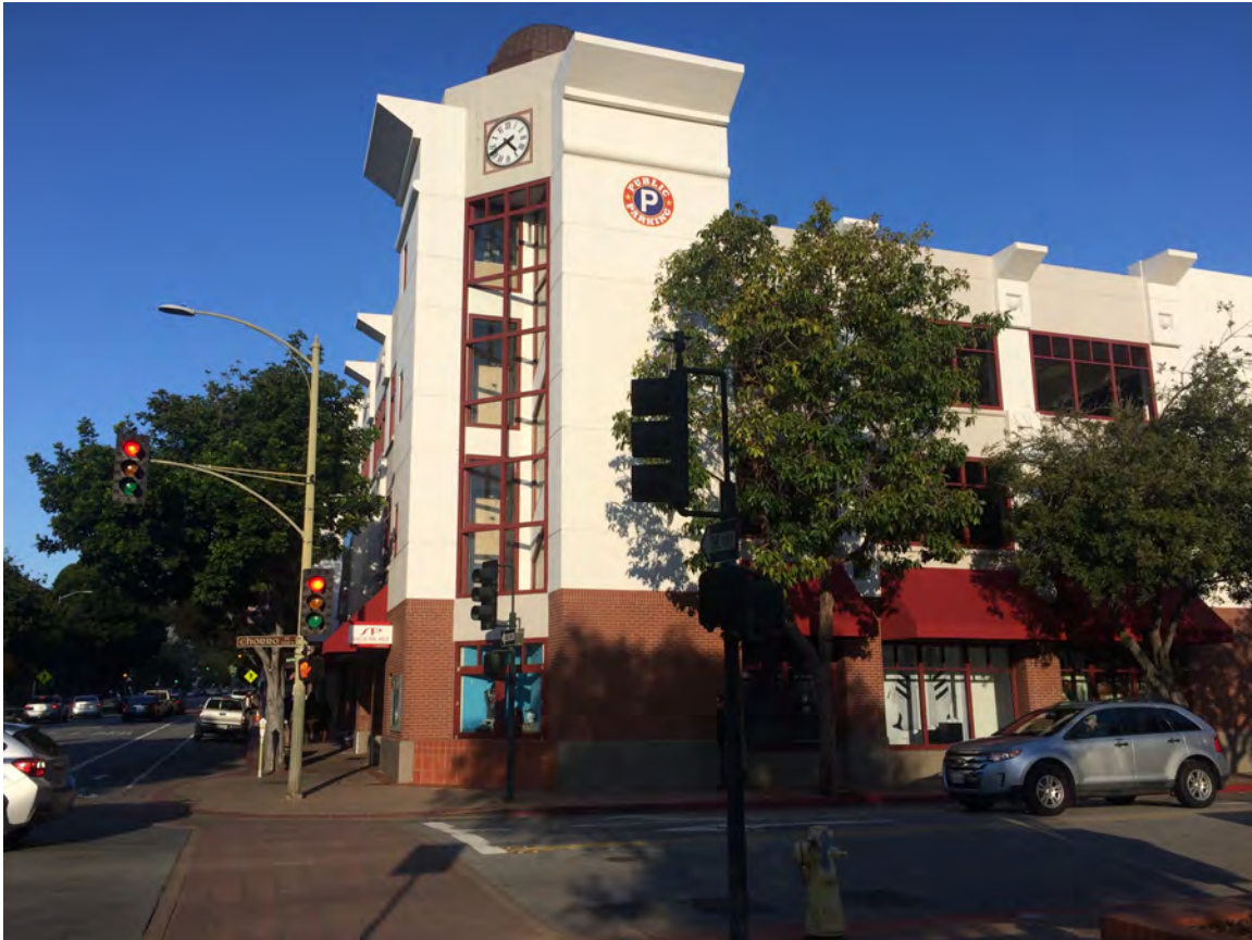
Figure 4.3 – 2: Even parking garages can be screened from public view by being wrapped in other buildings, or having the ground floor adjacent to the main corridor feature commercial space.
