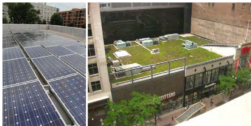
Figure 4.2 – 21: Rooftops can be used as a location for solar arrays to help offset energy needs (left), or for green roofs (right), which help reduce energy needs for heating/cooling. (Creative Commons, Attributive-ShareAlike, https://www.flickr.com/photos/arlingtonva/6284322776 ; Creative Commons, Attributive, https://www.flickr.com/photos/andrewzahn/4811639078 )
