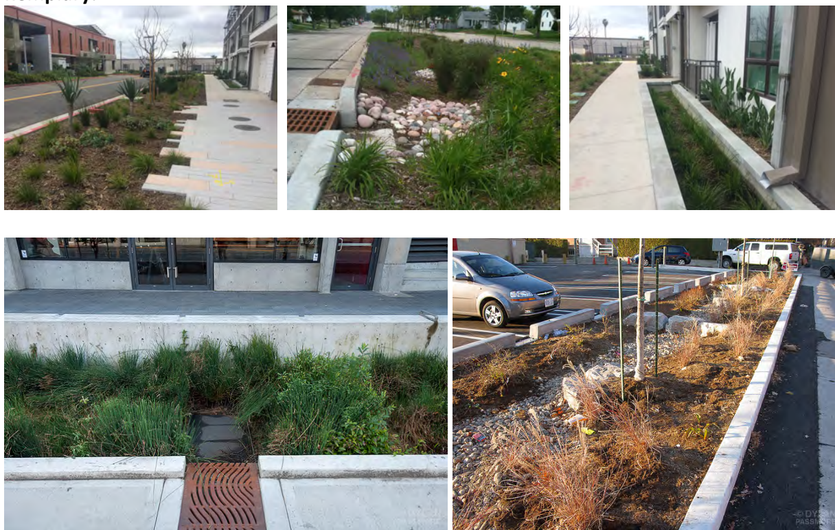
Figure 4.4 – 3: Bioswales serve double as a way to control storm water runoff, as well as landscaping areas for streets. (Creative Commons, Attributive, https://www.flickr.com/photos/87297882@N03/8183599860 ; Creative Commons, Attributive-Noncommercial, https://www.flickr.com/photos/dylanpassmore/7559851982 ; Creative Commons, Attributive-Noncommercial, https://www.flickr.com/photos/dylanpassmore/6939383075 )
