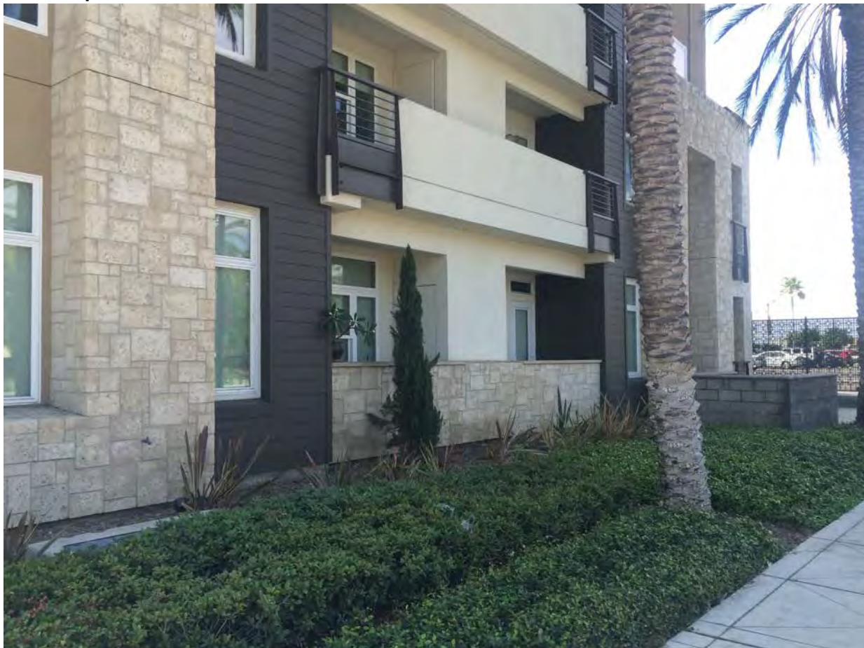
Figure 4.2 – 3: These units, although setback from the street, and somewhat screened with landscaping are at-grade with the street. This allows all passerby to peer into an otherwise private apartment.
