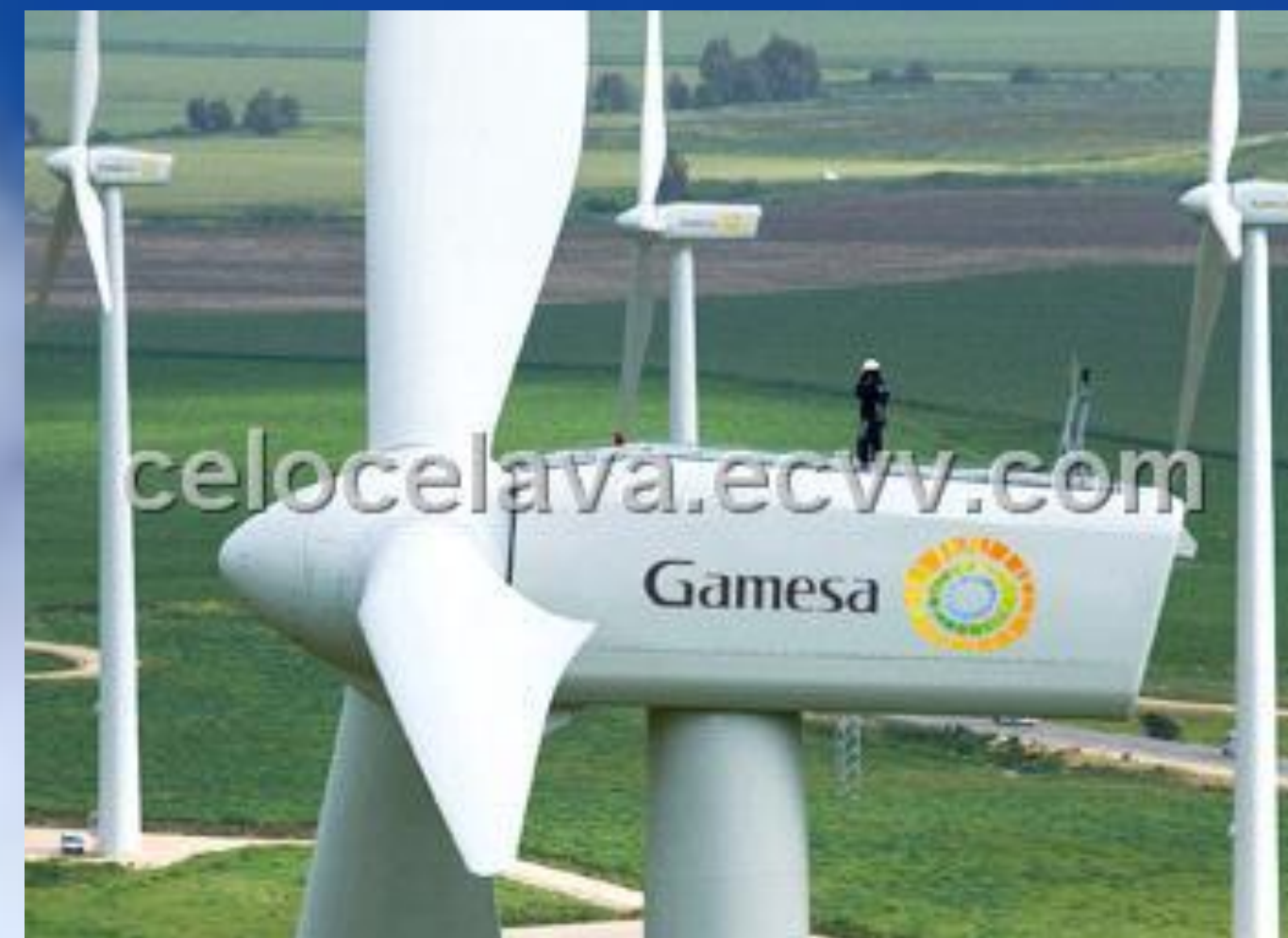
Utility scale wind turbines are big, up to seven megawatts. (Note the person.)
