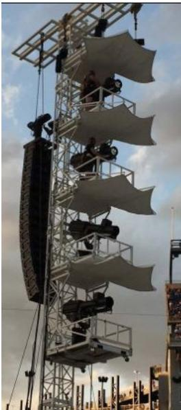
*Figure 3: WorldWired Tour delay tower with four spotlight platforms*
