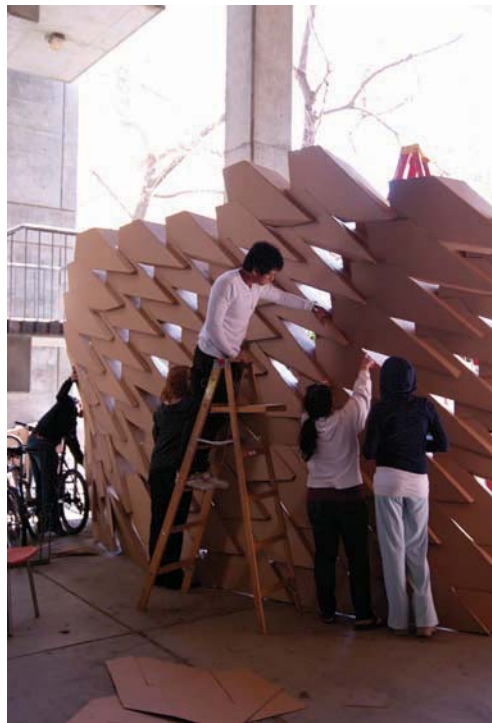
Final installation on Sunday afternoon. At their discretion, the students assembled and re-assembled the entire installation twice testing out configuration variations and location as the open ends required a fixed point to attach to. Like a tensile fabric, the elliptical shape took on a nice anticlastic curve.
