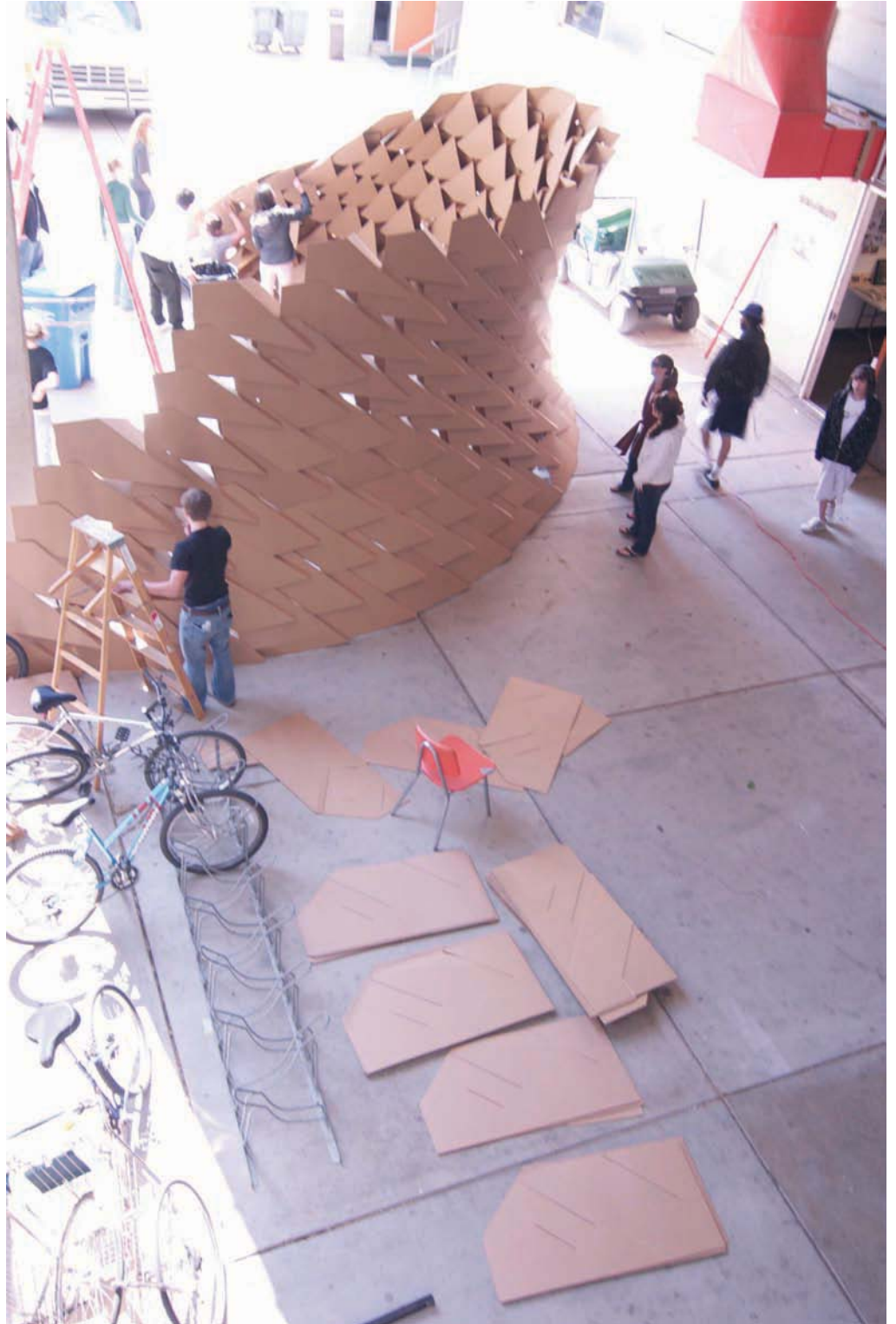
Scalar Shifts: refined model hand cut from ▲ 2d cut files studying openings in system. Further developed cut file with variations ▼ and full scale assembly from flat pieces. ▶
