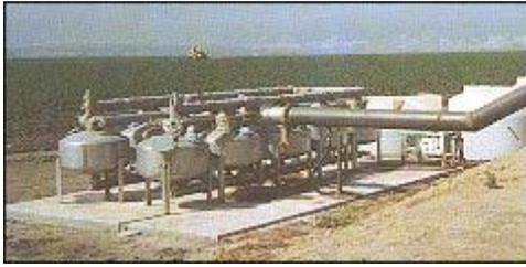
**Injectors should be installed upstream from filters**
