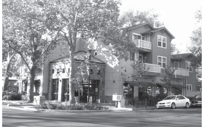
Figure 7. Mixed use condos. Downtown, Davis. (photo courtesy The Local Government Commission)
