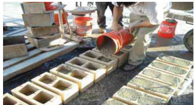
Figure 2: Grout Placement in Concrete Masonry Unit Cells
