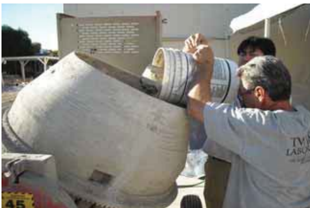
Figure 1: Adding Grout Materials to a Mechanical Mixer
