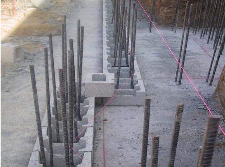
Figure 6: CMU Reinforcement Placement
