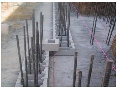
Figure 6: CMU Reinforcement Placement
