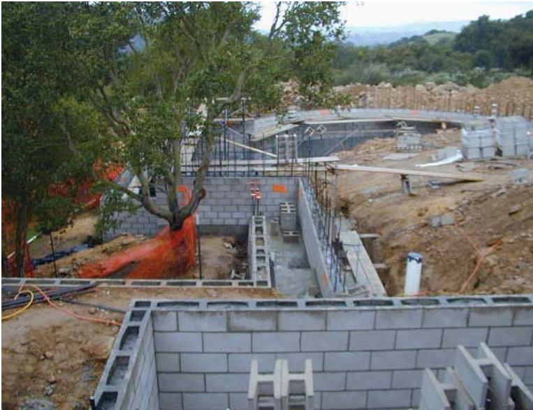
Figure 7: CMU wall showing grouting
