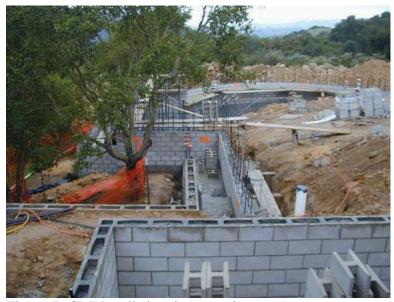
Figure 7: CMU wall showing grouting
