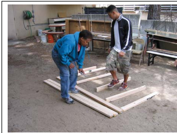
Fig. 2a: Laying Out the Wall
