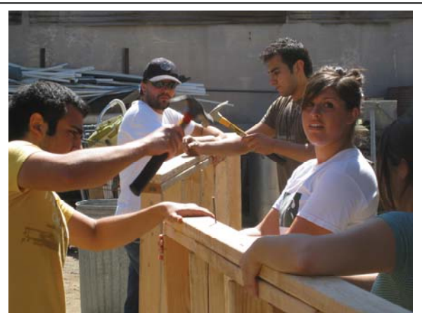
Fig. 5: Double Top Plate Nailing
