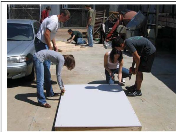
Fig. 6a: Applying Sheathing
