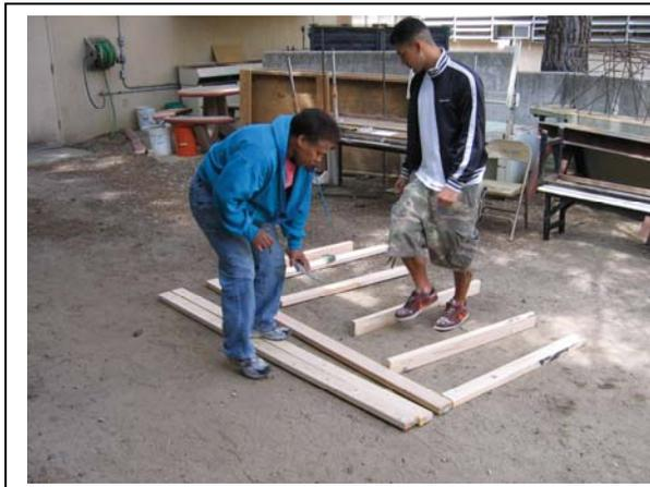
Fig. 2a: Laying Out the Wall
