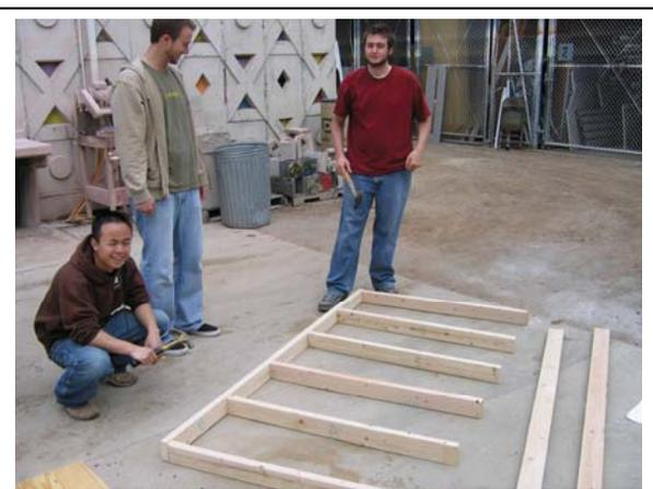
Fig. 2b: Laying Out the Wall
