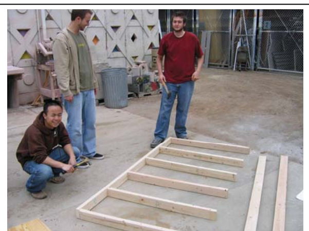
Fig. 2b: Laying Out the Wall
