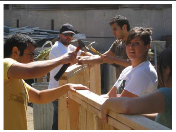
Fig. 5: Double Top Plate Nailing
