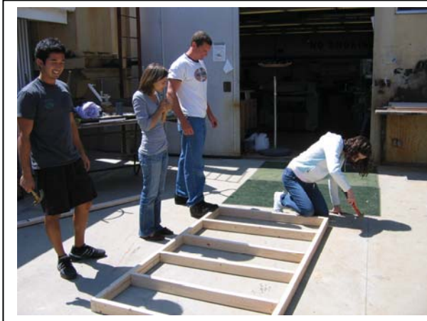
Fig. 4b: Wall Framing
