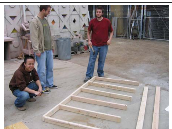
Fig. 2b: Laying Out the Wall
