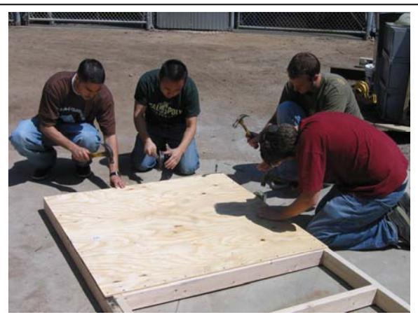
Fig. 6: Applying Sheathing
