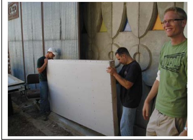
Fig. 8: Bolting the Wall to the Foundation
