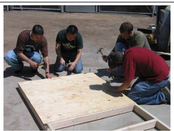
Fig. 6: Applying Sheathing
