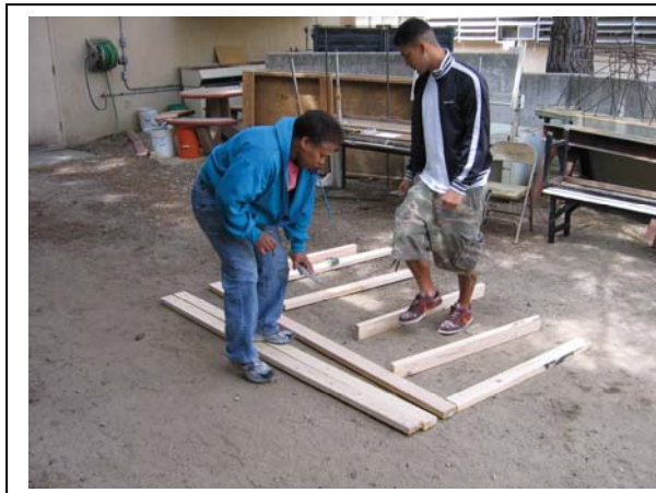
Fig. 2a: Laying Out the Wall
