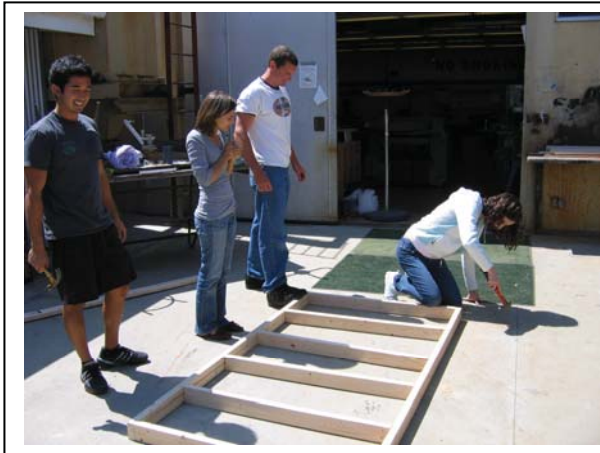
Fig. 4b: Wall Framing
