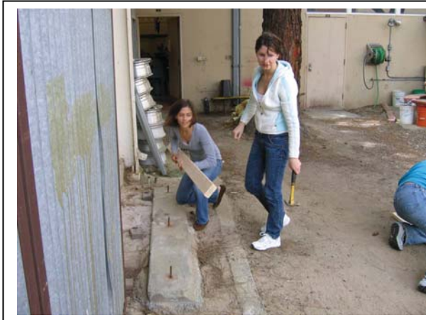
Fig. 3: Measuring for Anchor Bolts
