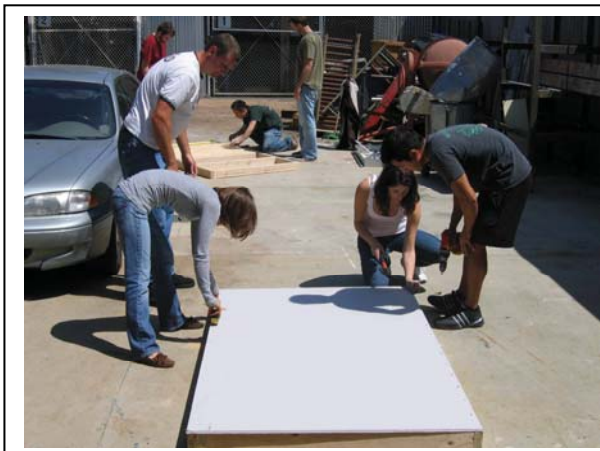
Fig. 6a: Applying Sheathing
