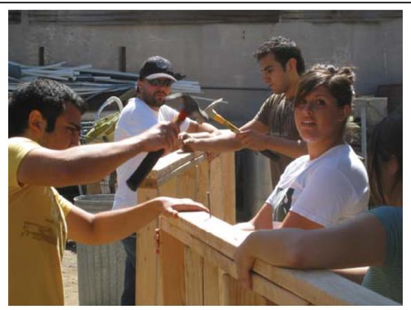
Fig. 5: Double Top Plate Nailing
