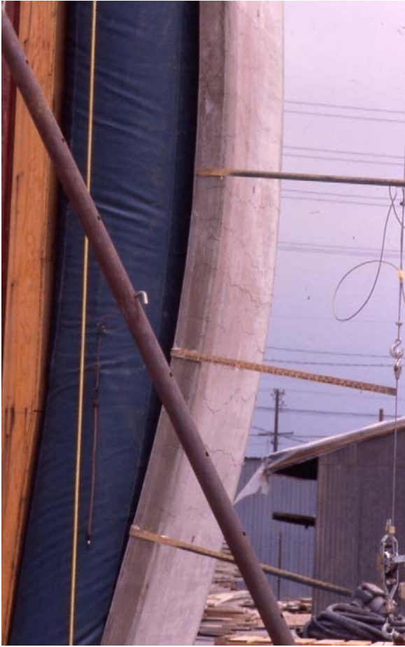
Fig. 4 – Test Panel Showing no Instability
