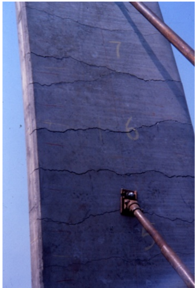
Fig. 5 – Test Panel Showing Cracking Pattern
