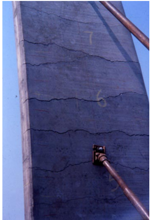
Fig. 3 – Test Panel Showing Cracking Pattern
