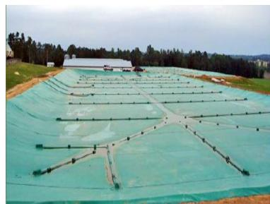
Figure 3 Covered lagoons have a flexible cover where the methane is collected and it's piped into a combustion device. (Agstar, 2010)
