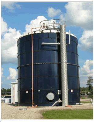
Figure 10 is an image that shows a fixed film digester. (AgStar. gov, 2010)
