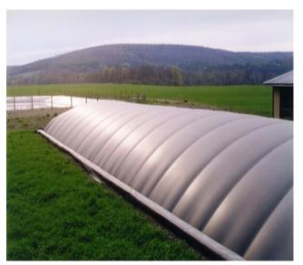
Figure 5 This figure shows the plug flow digester system. (AgSTAR, 2010)
