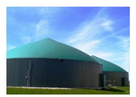
Figure 7 This is an image of a complete mix digester. (AgStar. gov, 2010)
