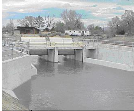
Figure 2. Completed installation of new check structure
