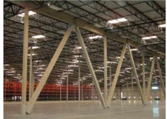
*Figure 1: Large HSS shapes have been common in braced frames in the seismically active western United States. Expanding the scope of ASTM A500 will allow use of these shapes that already comply with the new seismic compactness requirements.*
