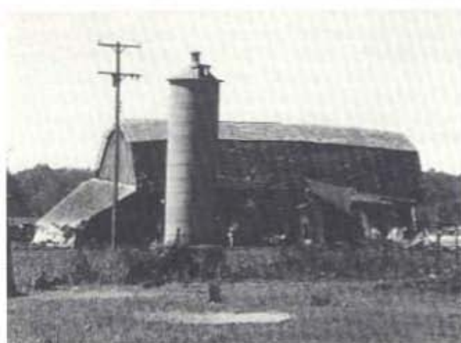
Figure 4: Silo constructed of stackable prefabricated concrete rings.
