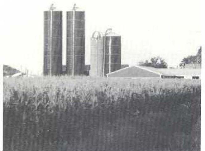
Figure 7: Multiple Harvestore silos on a prosperous farm.
