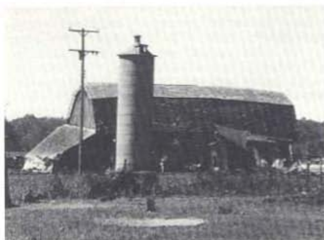
Figure 4: Silo constructed of stackable prefabricated concrete rings.
