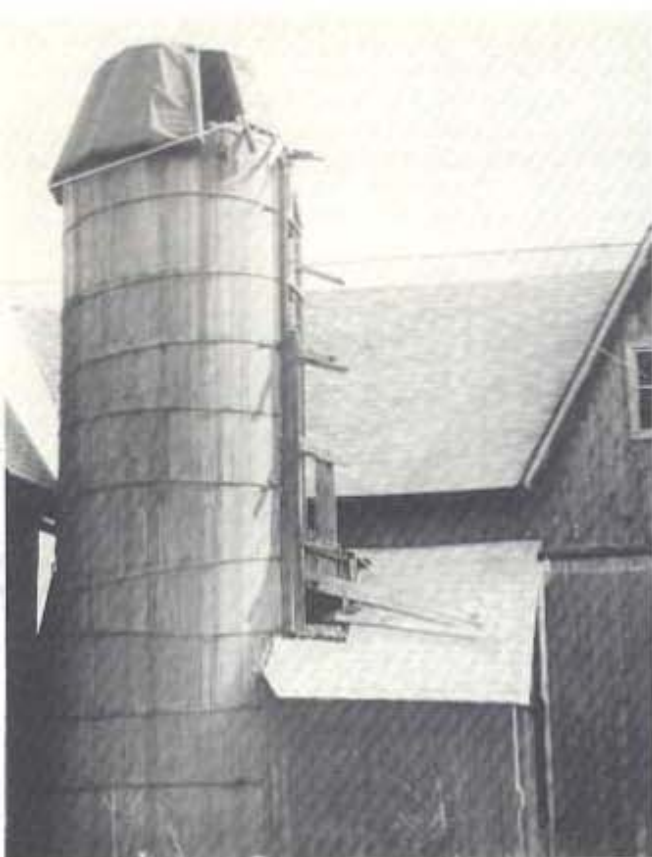
Figure 3: Wood stave silo.
