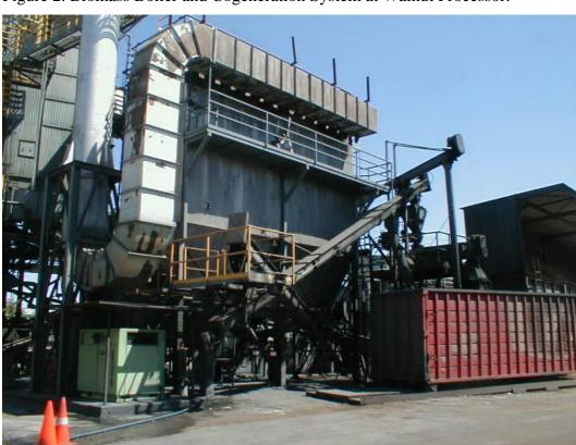
Figure 2. Biomass Boiler and Cogeneration System at Walnut Processor.
